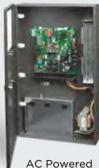
AC Powered Control Box
