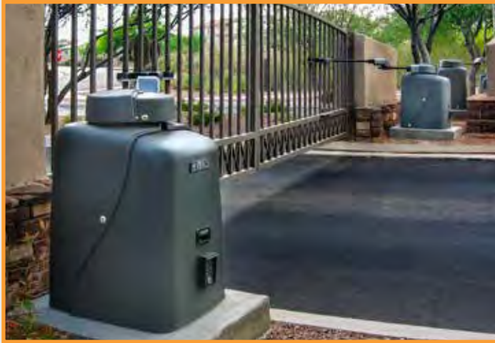
Dual gate configuration includes non-colliding overlap feature.
