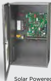
Solar Powered Control Box
