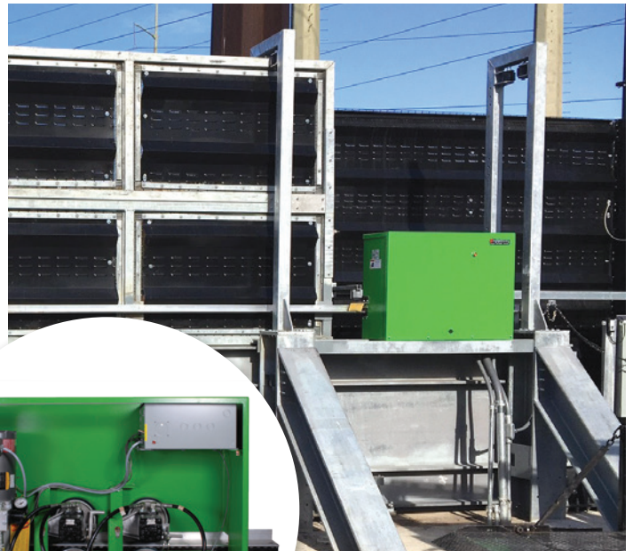
SlideDriver 200 operates crash gate at power substation
